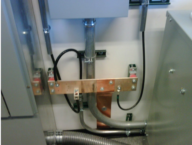
Bulkhead ground for coax cables
